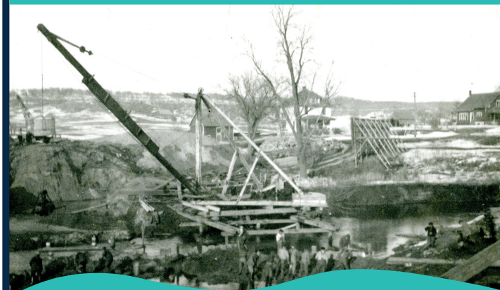
▲ Silver Lake dam construction, 1936.
