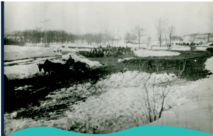
▲ Digging out and grading of Silver Lake, ca. 1931.
